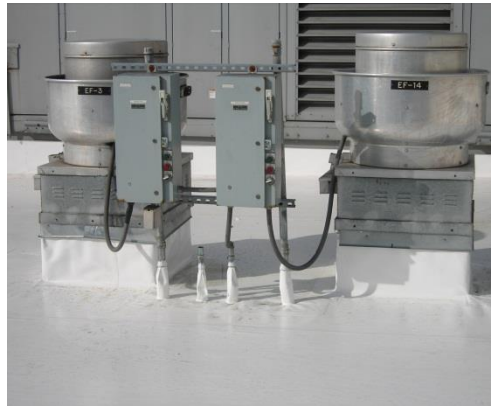
CURBS & PIPE STACKS
