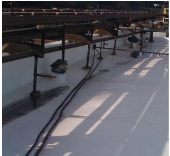
RE-ROOFED WITH DURO-LAST
