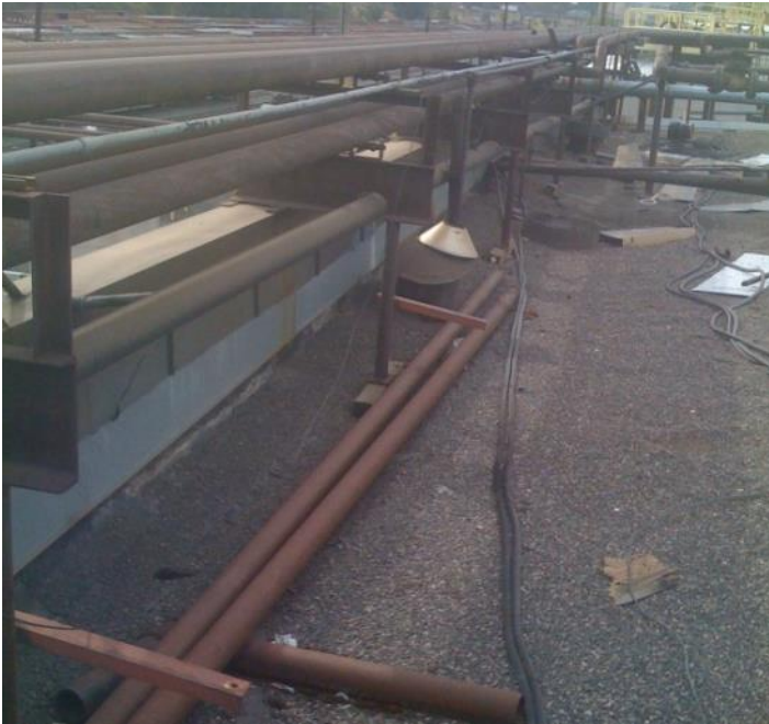
EXISTING BUILT-UP ROOF...
