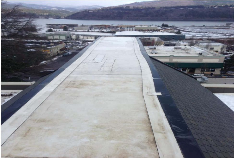
ROOF HAS PATCHES AND EDGE DETAIL ISSUES
