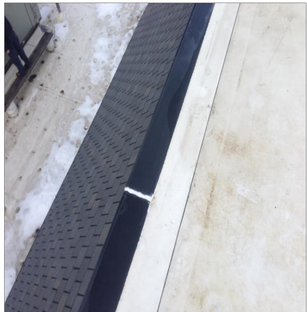
METAL EDGE DETAIL IS FAILING
