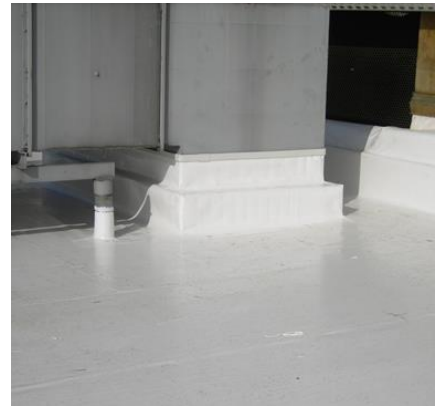
DOUBLE CURB & EXPANSION JOINT
