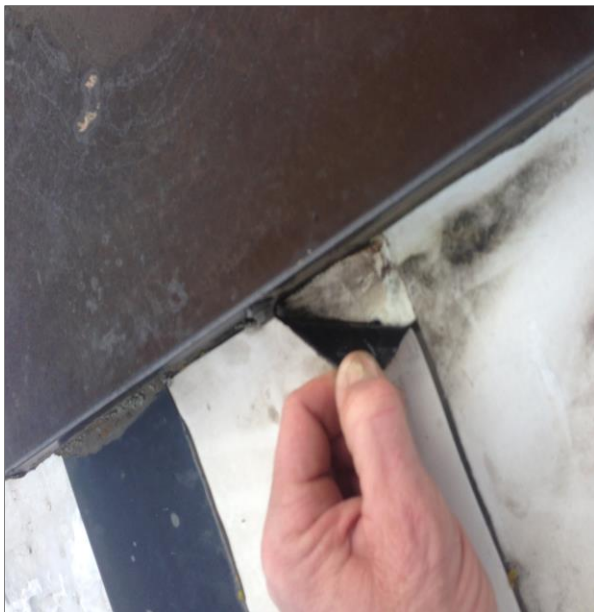
TAPE IS NOT PROPERLY ADHERED
